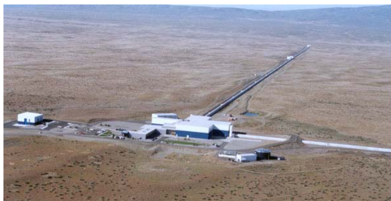
Figure I-5. LIGO Observatory Facility.
